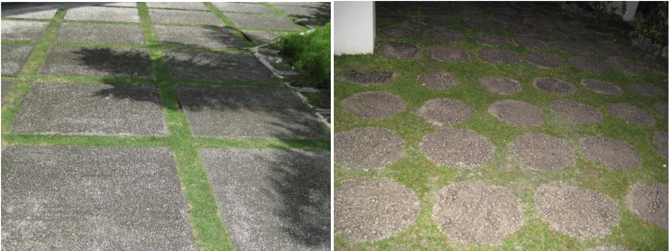
Figure 3: Example of a concrete pavement mixed with grass to create pervious areas. Picture taken at Sagicor’s office in Town A on 24/08/12 (LHS) and a local residence in Town A on 24/08/12.
